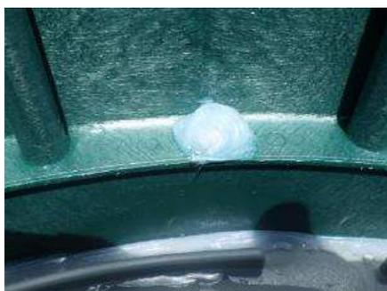
**Apply silicone to the screw head to prevent water penetration.**
