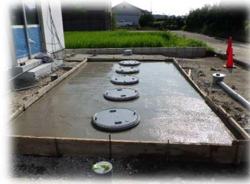
Step 15: Be sure to pitch final grade away from covers to sweep surface water away from system.
