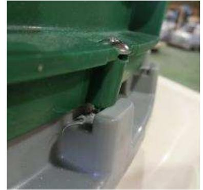
**Tuf-Tite Risers. Align riser screw holes with molded "frame block" and screw tight. Maximum screw length is 1 ¼"**
