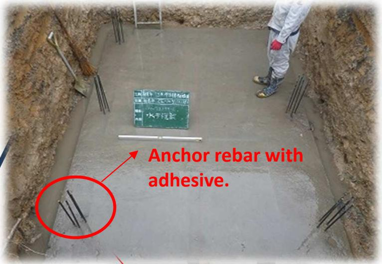
**Adhesive anchoring installation structure**
