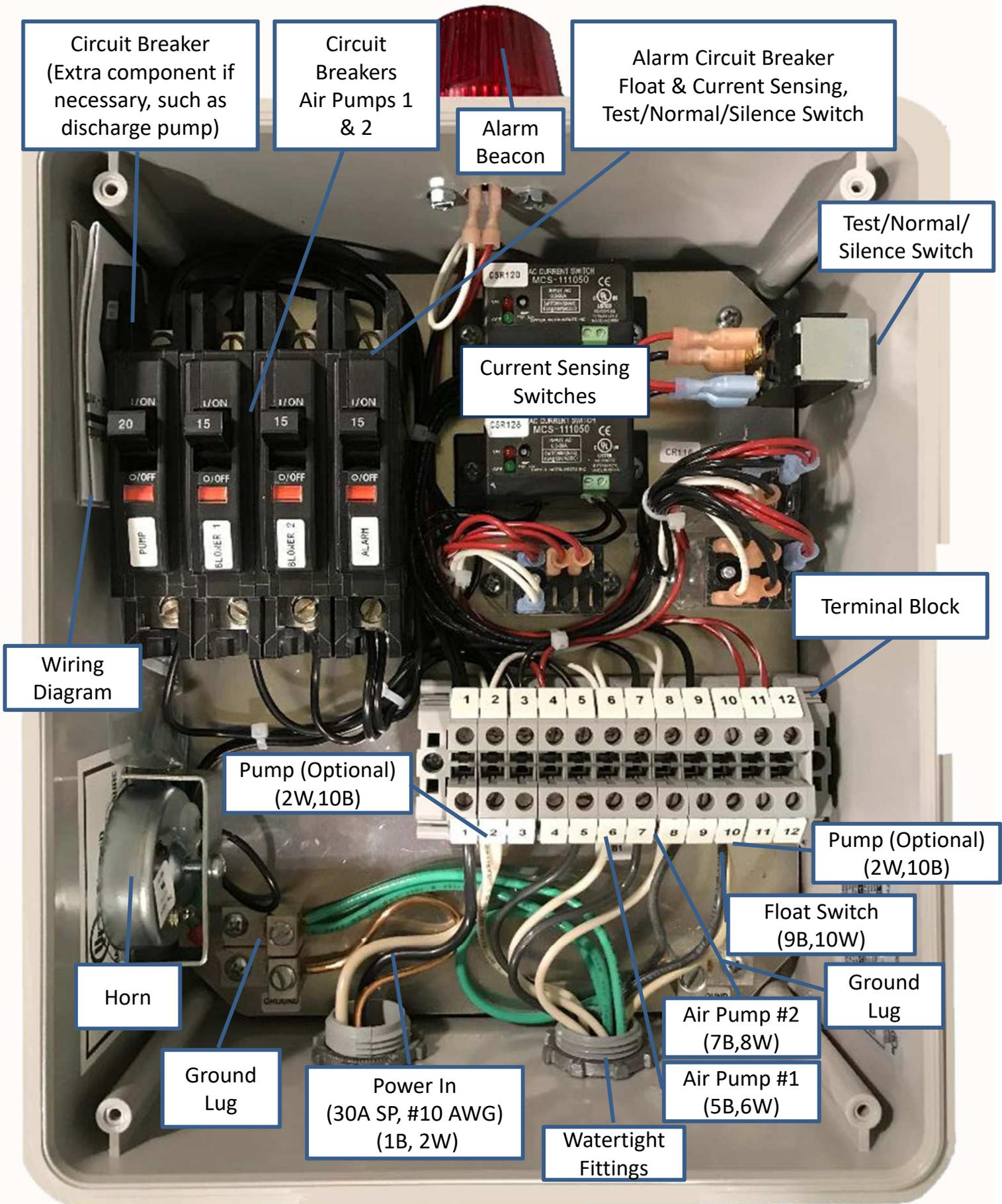
**Important note for all panels with current sensors.** Current sensors have an adjustable range of .5-50 Amps. Sensitivity is controlled with a screw dial. If screwed down to "Low" it would be set to monitor for .5 Amps. If the screw is rotated to "High" it would be set to monitor for 50 Amps.
